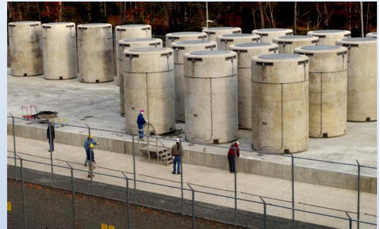
Connecticut Yankee - Spent Nuclear Fuel Rod Storage
