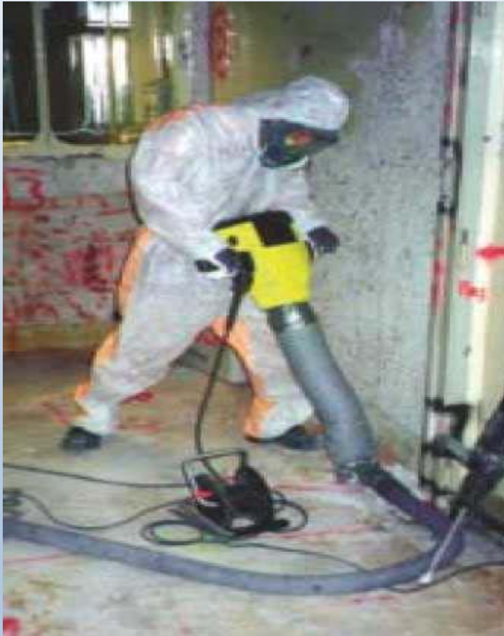
Contaminated areas are drilled away and disposed
