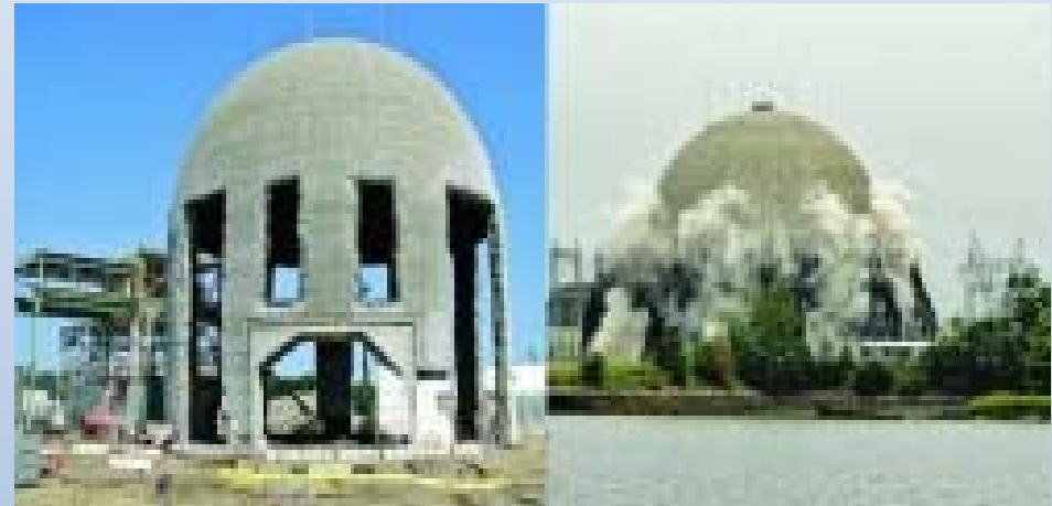
Demolishing Maine Yankee Containment Dome
