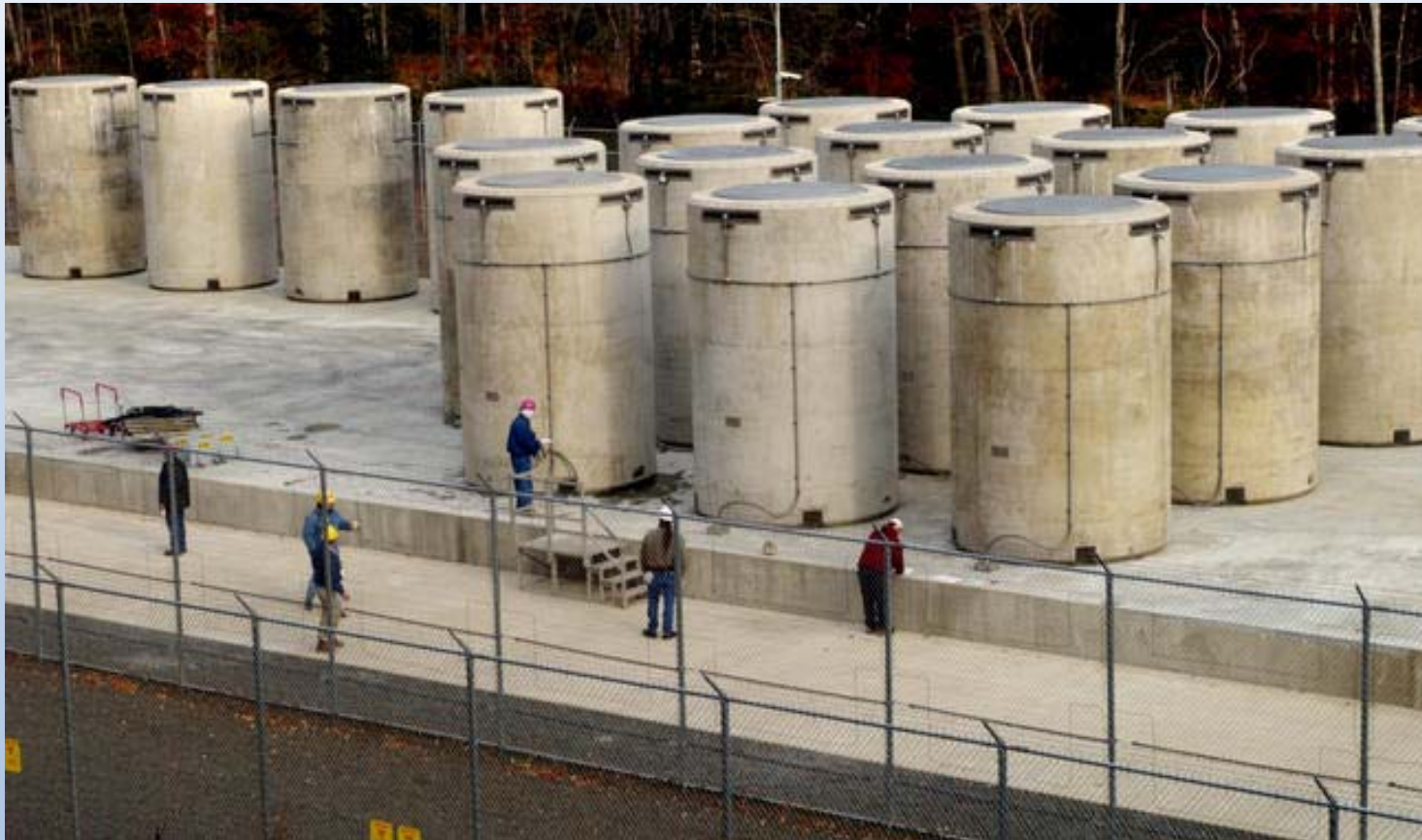
Connecticut Yankee - Spent Nuclear Fuel Rod Storage in Vertical Concrete Vessels. Facility cost: $31.6 Million (USD)
