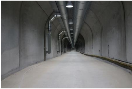
Fig. 1. Underground Research Tunnel at the Korea Atomic Energy Research Institute (KAERI).
