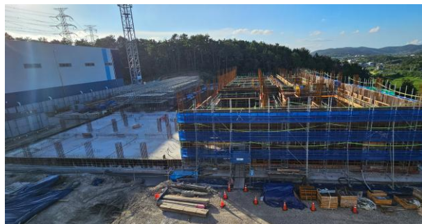
Fig. 2. Demonstration/Analysis Building Under Construction.
