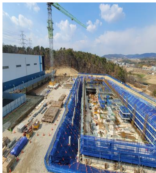
Figure2. Construction photograph of demonstration analysis building
