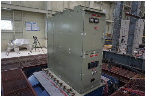
Fig. 3. Experimental shaking table setup of cabinet equipment (switchgear) for seismic fragility assessment
