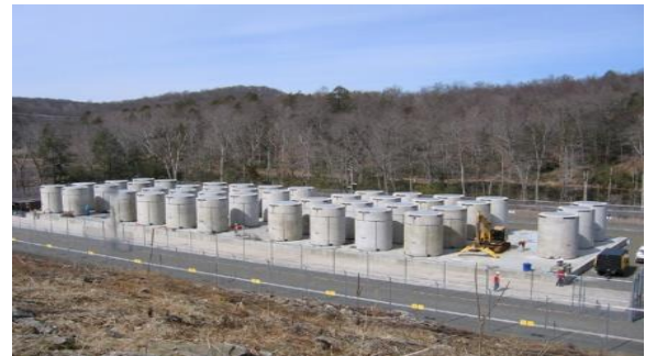
Fig. 1. Independent Spent Fuel Storage Installation (ISFSI)
