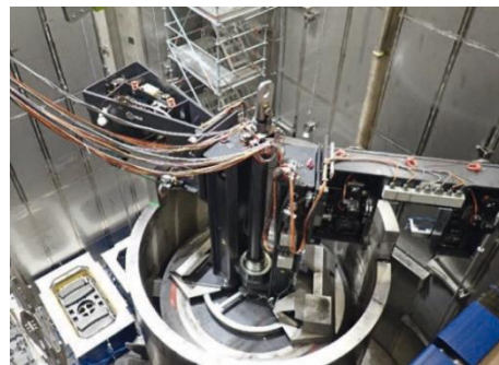
Fig. 3. “The Beast”, a bandsaw system working on RPV cylinder.
