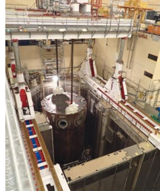
Fig. 2. Lifting the RPV out of its installation position.
