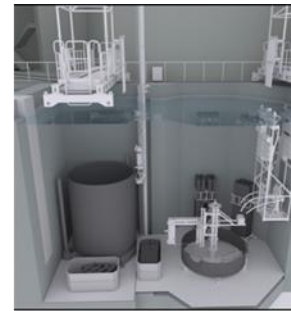
cutting of core shroud
