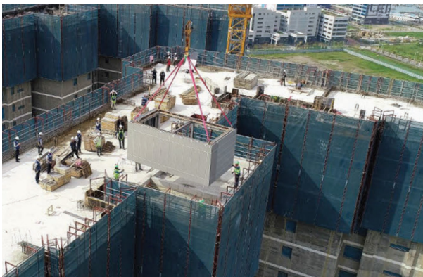
Fig. 4. Modular rooftop construction sequence [5]
