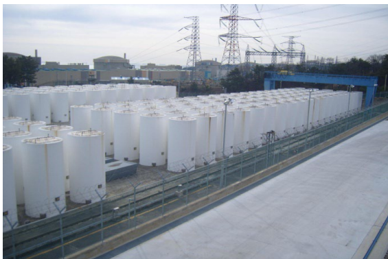
Fig. 1 Silo dry storage facility
