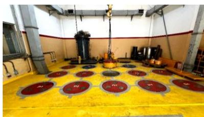
Fig. 1 Interim storage with underground cylindrical well
