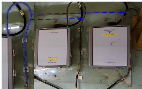
Fig. 2 Electric noise shielding tape attachment
