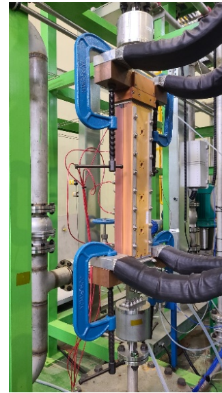
Fig. 1. Installed Test Section
