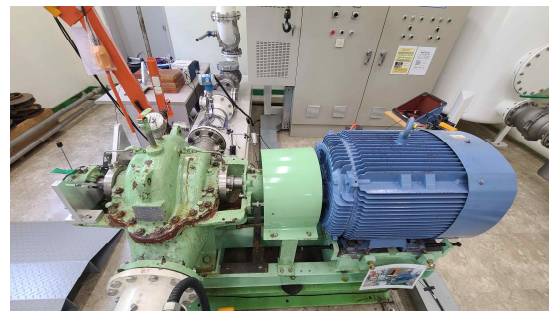
Fig. 1. Pump test bed for acquiring vibration data according to shaft misalignment
