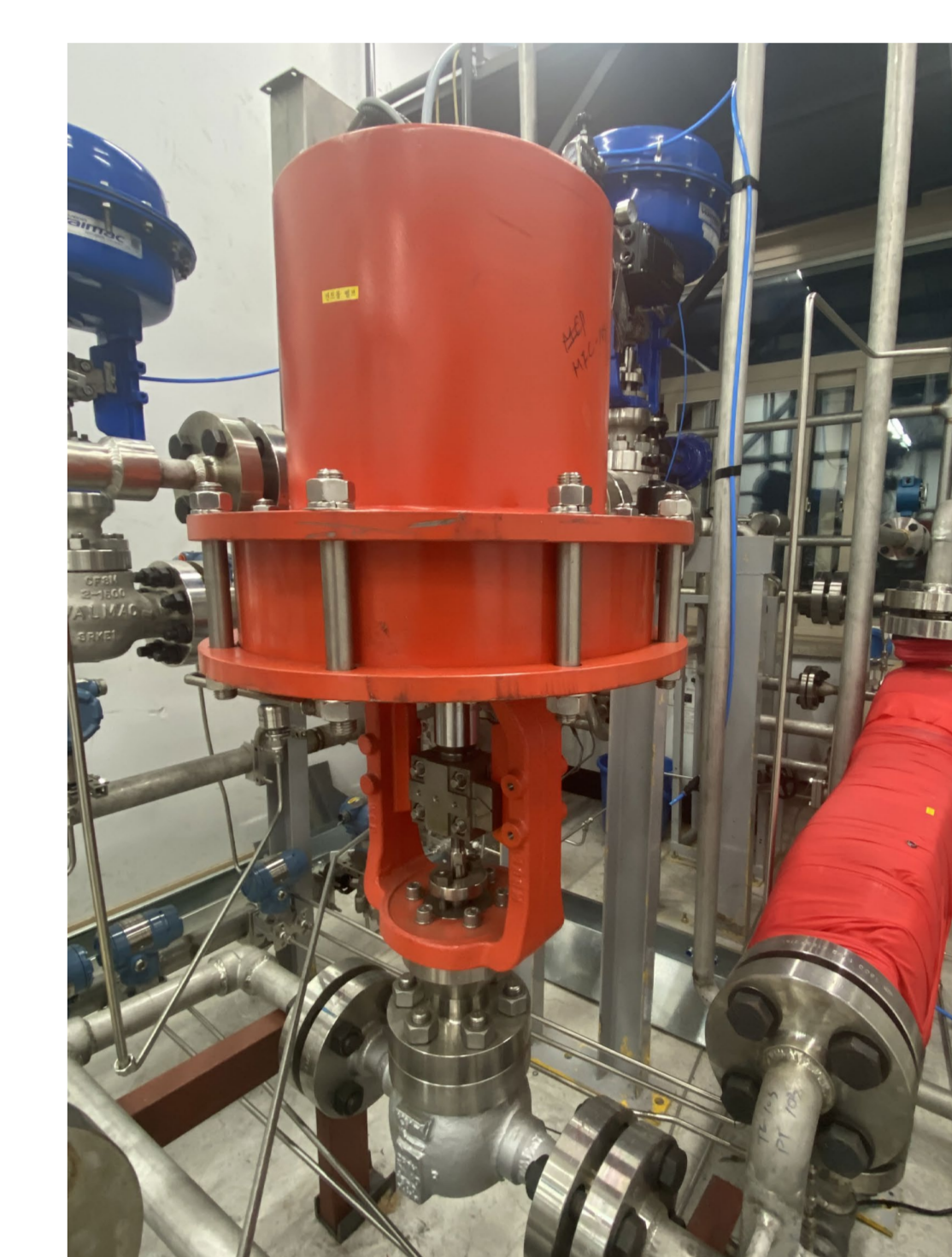
▲ Control valve for bypass control
