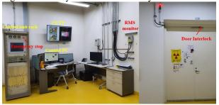
Figure.4 Layout of the interlock system
