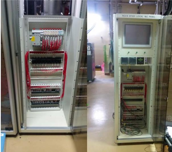
Figure 8. PLC Installation and Termination
