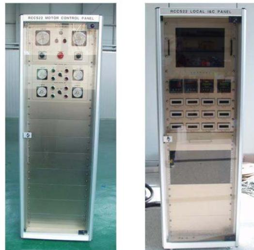
Fig. 3. RCCS motor control panel and local control panel.
