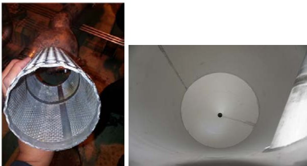
Fig. 3. Inspection results of the PWMS strainer and FRST inside after flushing.
