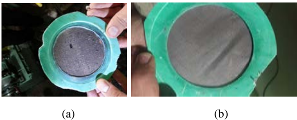
Fig. 2. Temporary strainer mesh and foreign materials of the PWMS pump inlet side. (a) after first flushing (#80), (b) after final flushing(#200).
