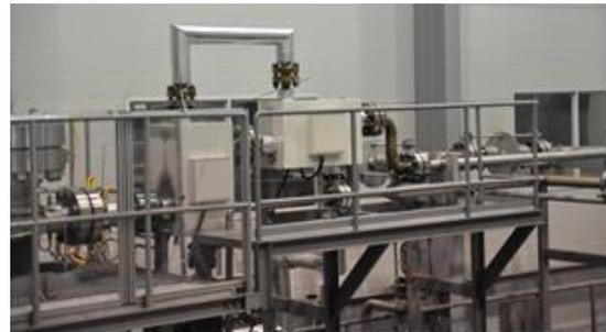
Fig. 3 Alloy617 Compact Heat Exchanger & 800HT Printed Circuit Heat Exchanger in HELP
