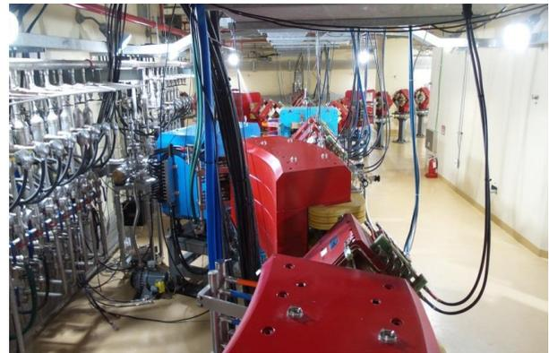
Fig. 10. Newly installed 45 degree bending magnets.
