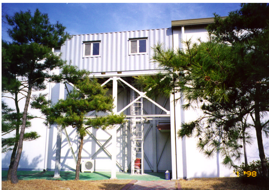
Fig. 4. Picture of constructed TOF facility
