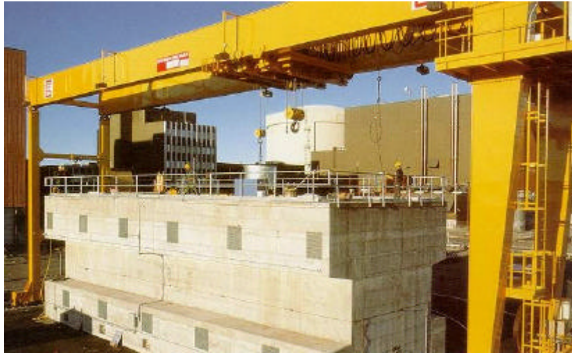
Figure 1. MACSTOR CANDU Spent Fuel Dry Storage Module in Operation
