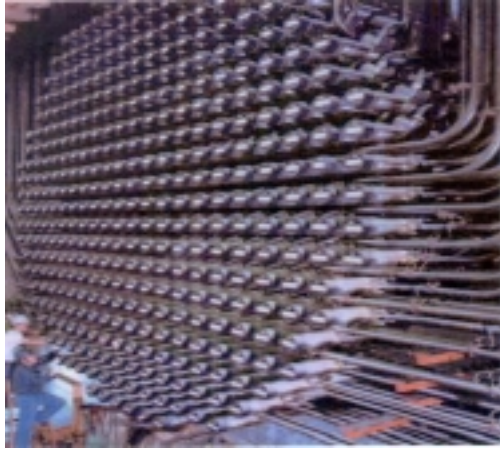
Fig. 1. Feeder pipes in CANDU reactor.
