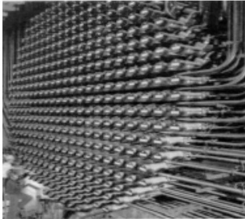
Fig. 1 Feeder pipes in CANDU reactor.
