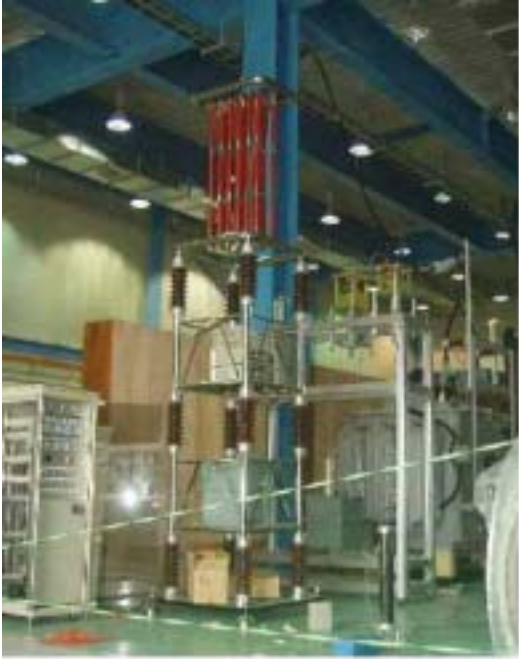
Figure 9. Test setup for opening switch
