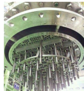
Fig. 1 Internal structures in the low plenum
