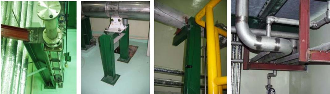
(c) Fixtures, Supports and Base Structures
