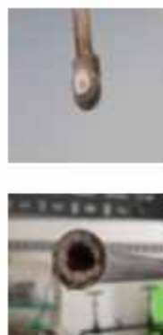
Figure 1. Sodium in pipes.
