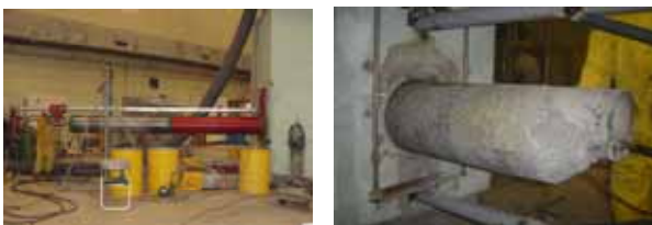
Figure 2. Beam port core boring and pulled out
