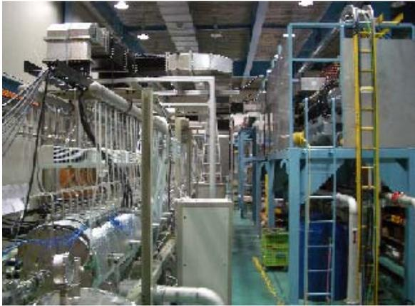
Figure 3: The installed HPRF system for the DTL
