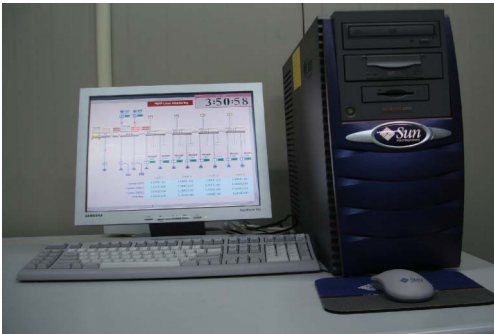
Figure3. PEFP control screen using EDM
