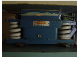
Fig. 1 Spring System of Drawing Ulchin 2 unit EDG
