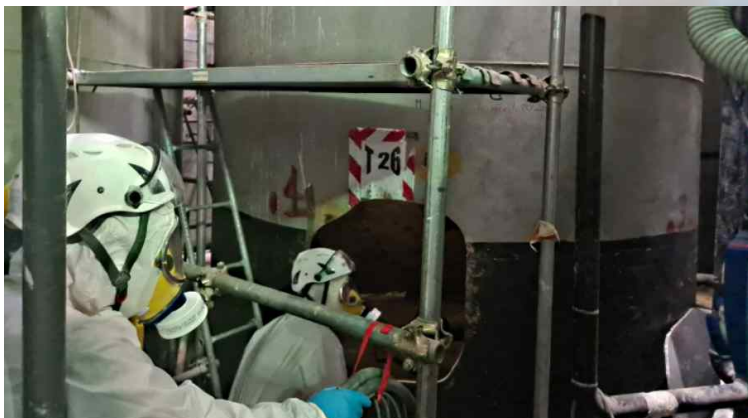
Removing the vessel head marks the start of the final phase of decommissioning of the boiling water reactor (Image: Sogin)
