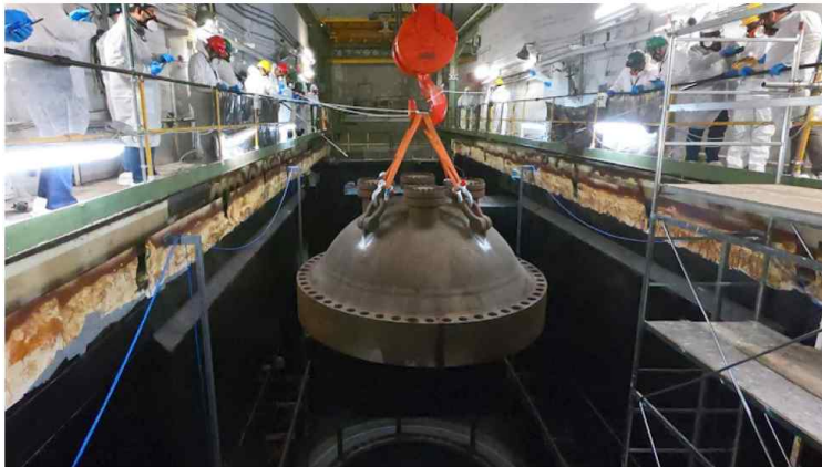
Removing the vessel head marks the start of the final phase of decommissioning of the boiling water reactor (Image: Sogin)
