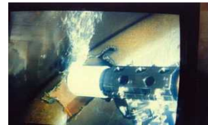
<Cutting of feed-water sparger>
