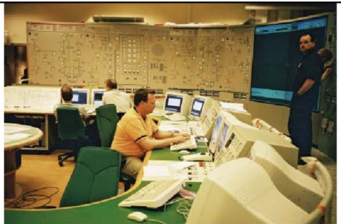
FIG. V-4b. Sweden's Oskarshamn unit 1 MCR after modernization
