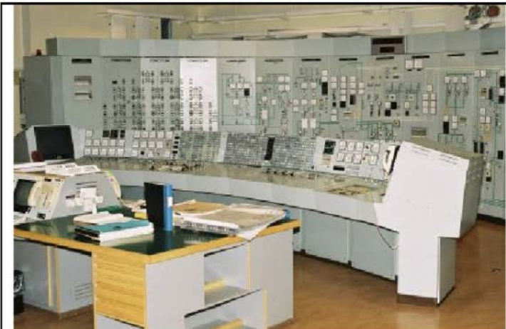
FIG. V-4a. Sweden's Oskarshamn unit 1 MCR before modernization in 2003
