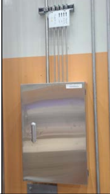
Plumbing of gas pipes for the detectors
