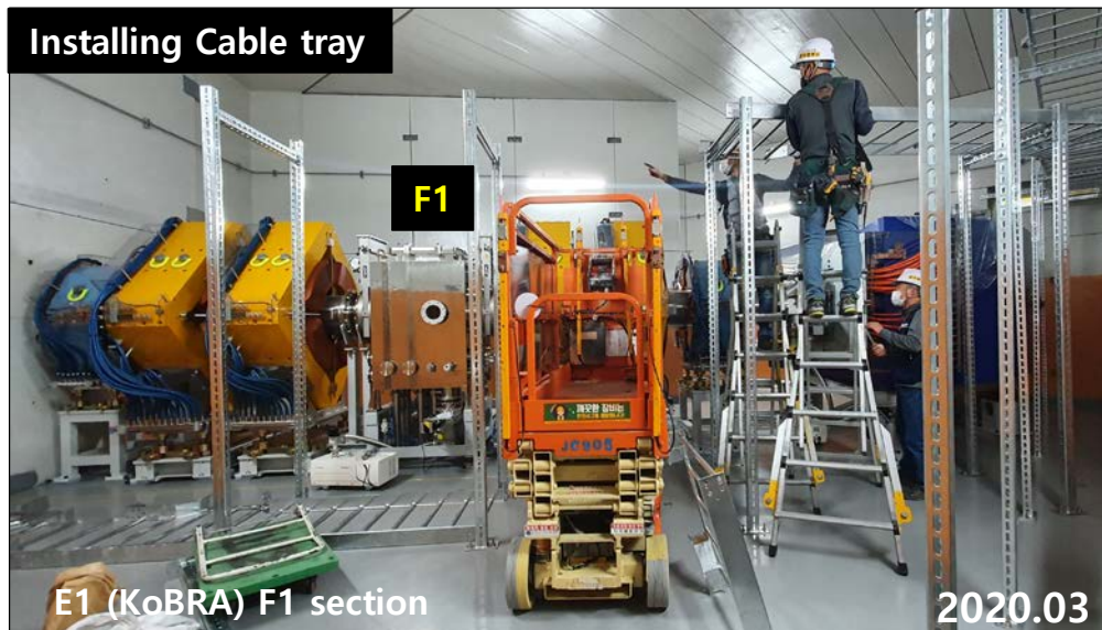
Power cable Wiring
