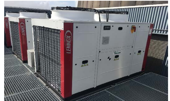
Chiller for Cryogenerator
