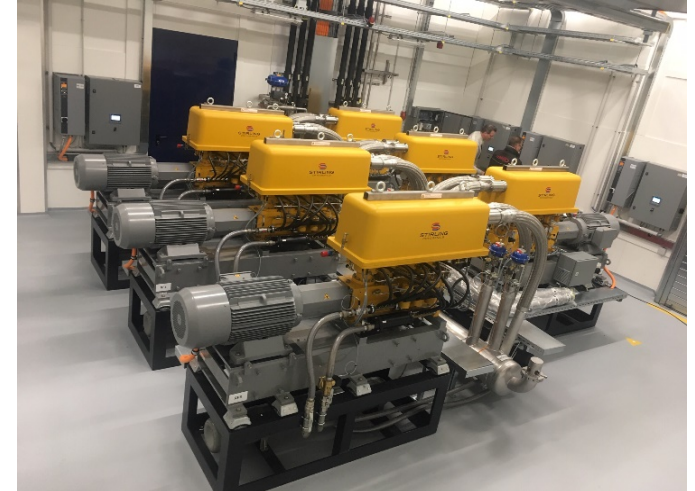
Cryogenerator (980W)
